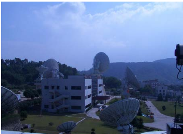
Guangdong Earth Station, Guangzhou, China
